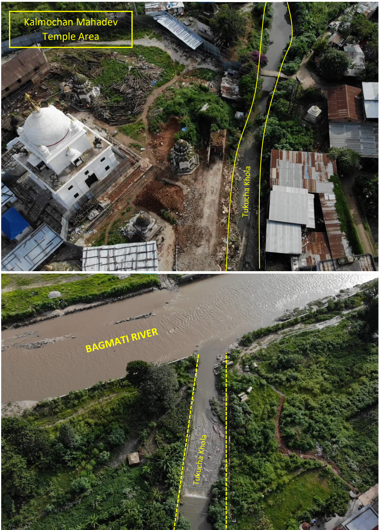
Figure 20 Segment X - Photos
