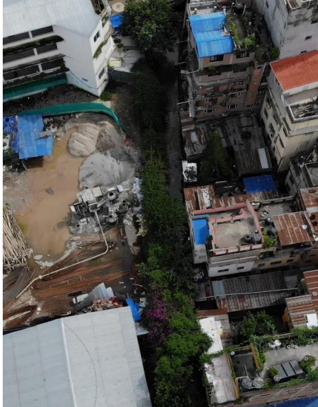
Figure 33 Existing Condition - Segment VI
