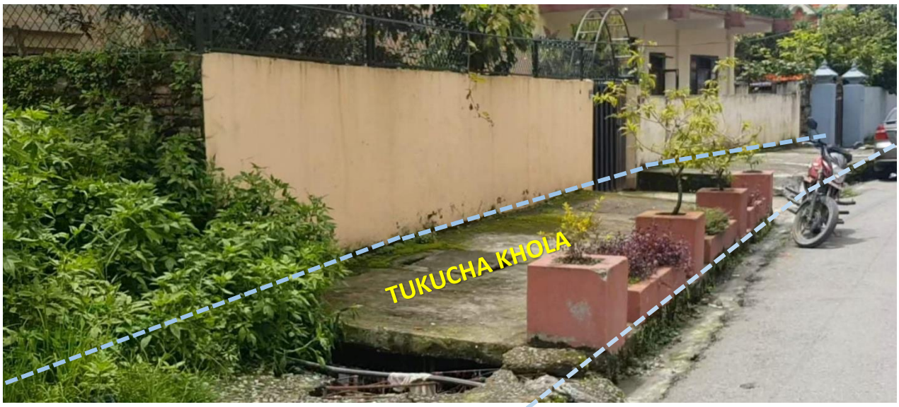
Figure 4 Segment I - Tukucha Khola covered with Slab
