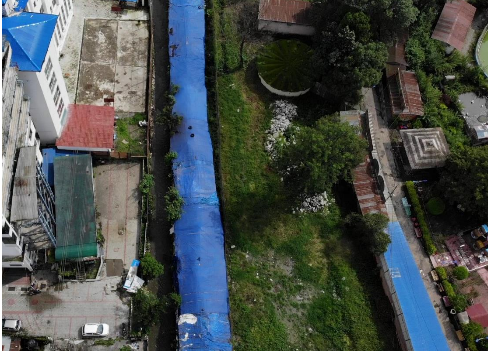
Figure 37 Existing Condition - Bhrikutimandap
