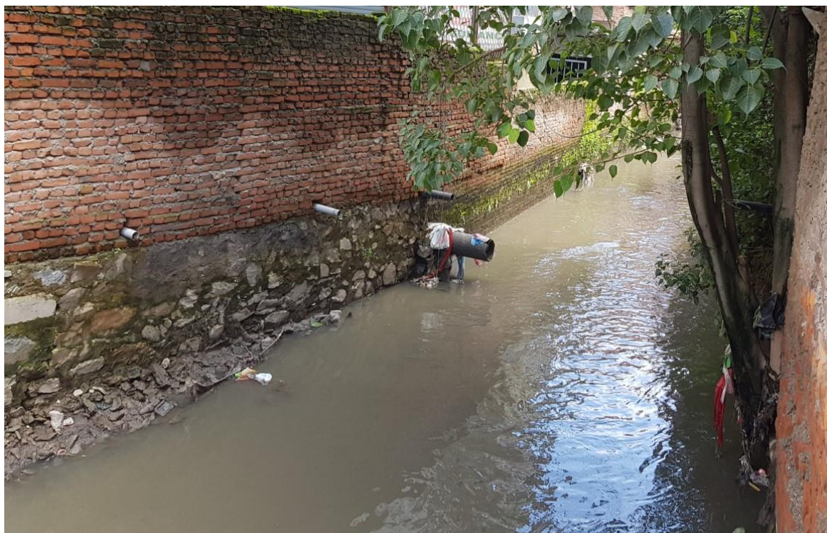
Figure 21 Sewers disposed to the river
