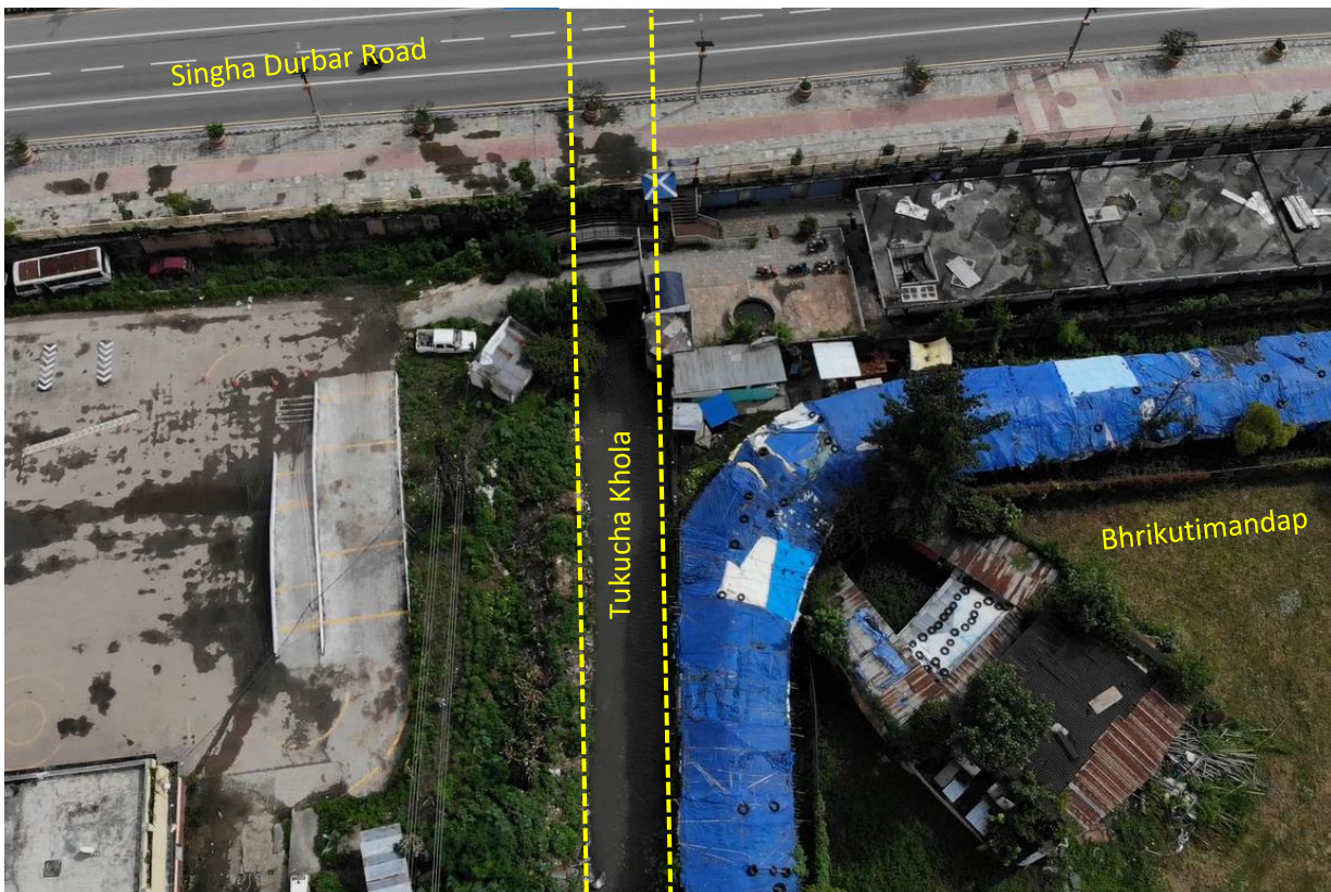
Figure 16 Segment VIII - Photos
