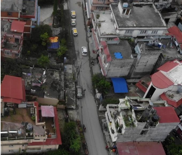
Figure 24 Existing Condition- Segment I
