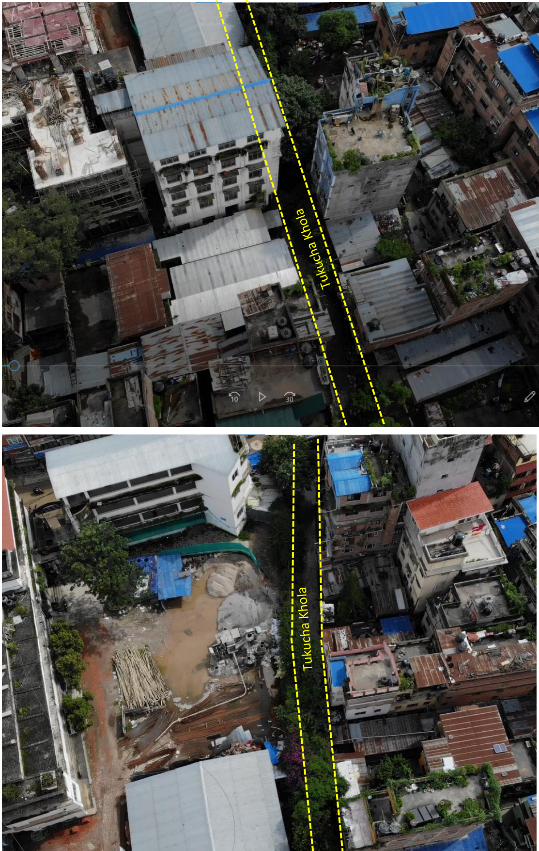
Figure 12 Segment VI - Photos
